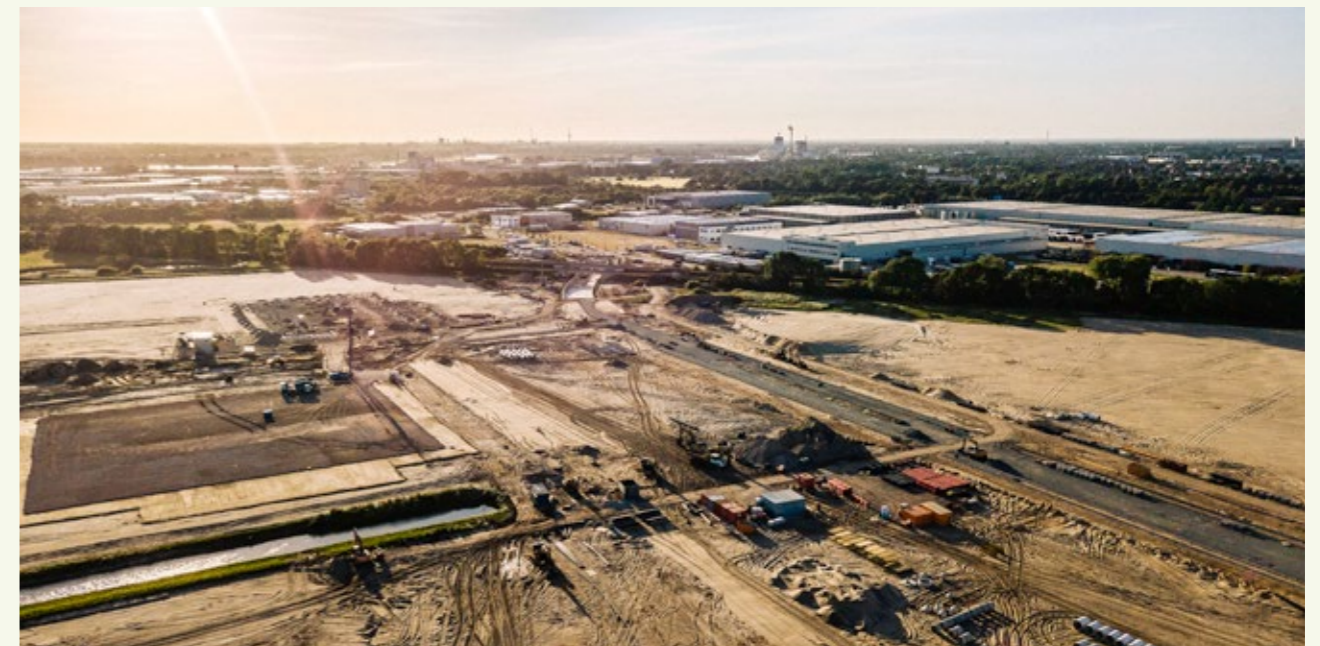
Developing the second stage of Hansalinie industrial estate
